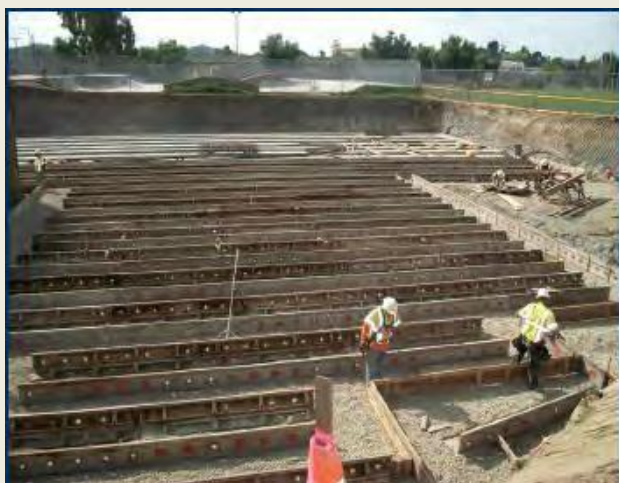
Storage tanks at Garvanza Park
