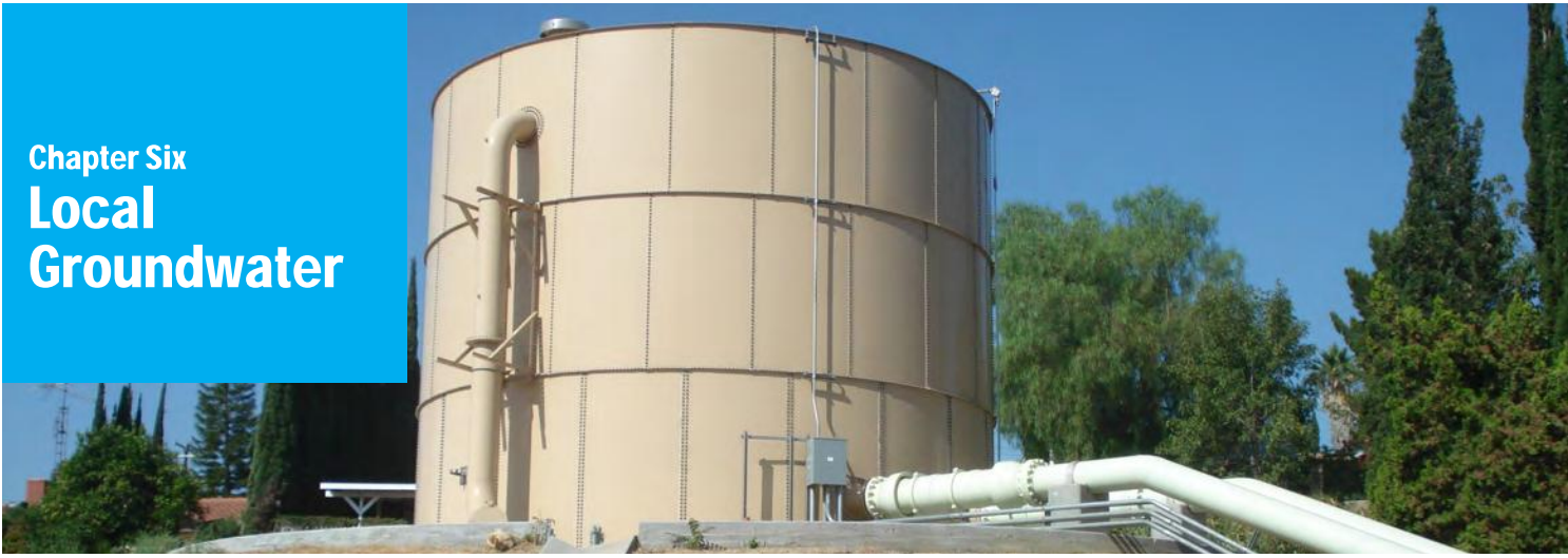
Mission Wellfield Water Tank
