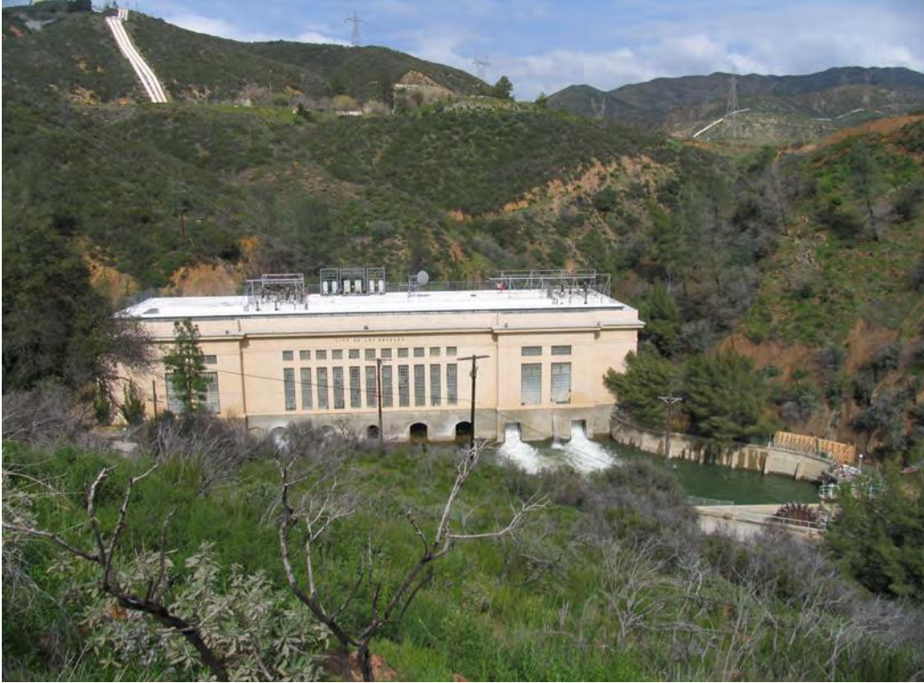
San Francisquito Power Plant Number 1
