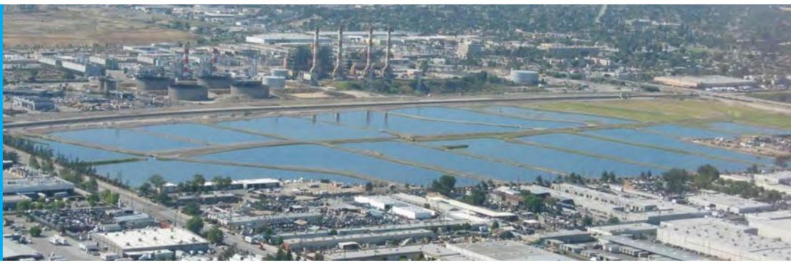
Hansen Spreading Grounds
