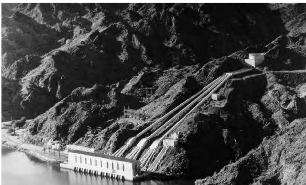
Colorado River Aqueduct Intake - Whitsett Pumping Plant at Lake Havasu, courtesy of Metropolitan Water District
